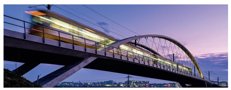
The jury of the critical German state prize for structural engineering explained its decision by stating that "as an innovation, the network arch bridge with carbon fibre–reinforced polymer cables with carbon hangers is an extremely successful example of civil engineering worldwide and provides formative answers to current issues in civil engineering".
